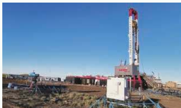
Drilling rig for new wells drilling
